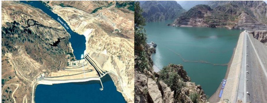
Figure 3: Daryan dam under construction on the Sirwan River in Iran.
